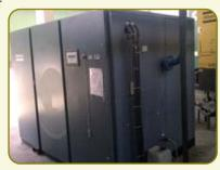
compressor with two new air compressors of 132 kW rating each in order to address the base load and peak load requirements in an energy efficient manner.
