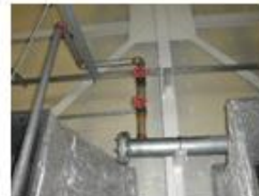
Riser pipe installed from above
