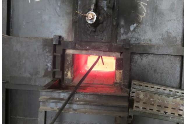
Re-heating furnace discharge door
