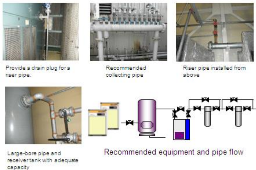
FIGURE 15: EXAMPLES OF RECOMMENDED PIPING
