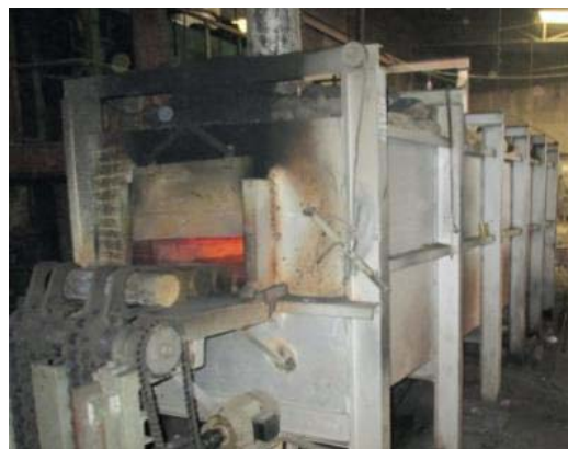
Figure 5.1: Re-heating furnace used in brass foundry units
