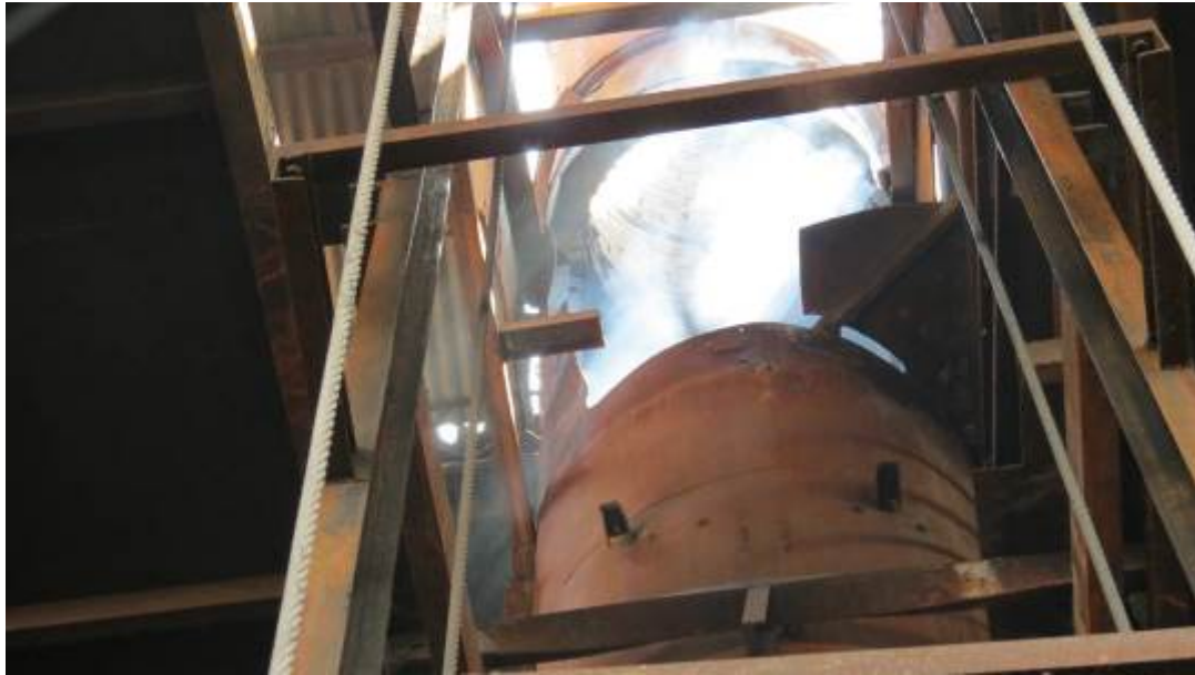
Figure 2.9: Upper portion of the cupola
