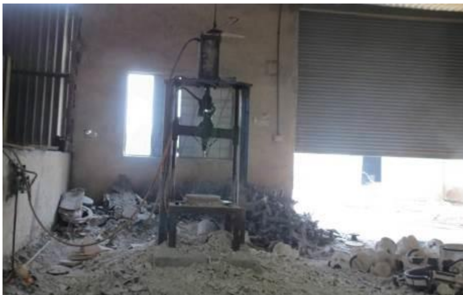
Figure 2.14: Removal of ceramic using pneumatic cylinder machine
