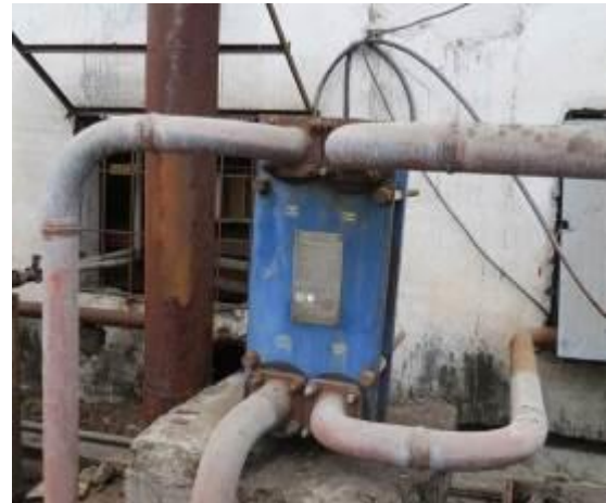
Figure 2.32: Pumps and plate type heat exchanger being used in the cooling circuit
