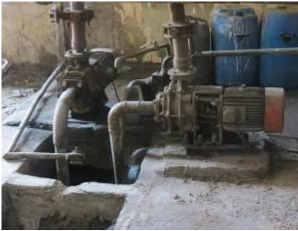
Figure 2.32: Pumps and plate type heat exchanger being used in the cooling circuit
