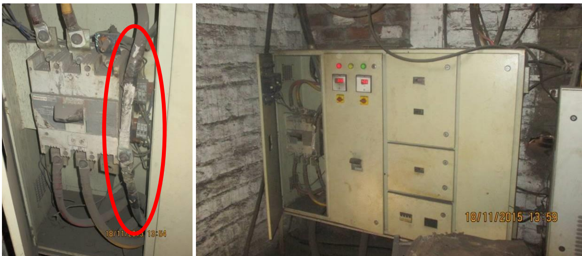
Figure 2.21: One phase (B- Phase) is direct/bypass
