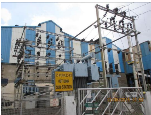
Figure 2.21: Pictorial depiction of transformers and power capacitor installed
