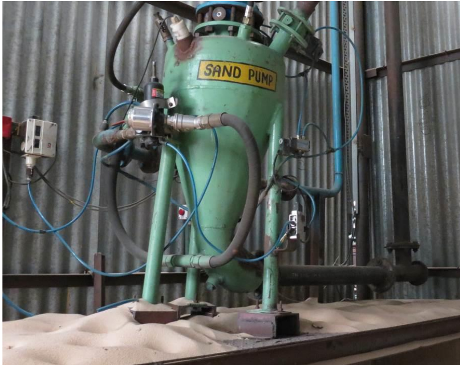
Figure 2.4: Sand mixer and pumping machine
