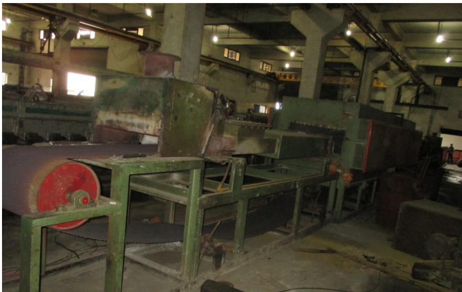
Figure 2.11: Machines being installed
