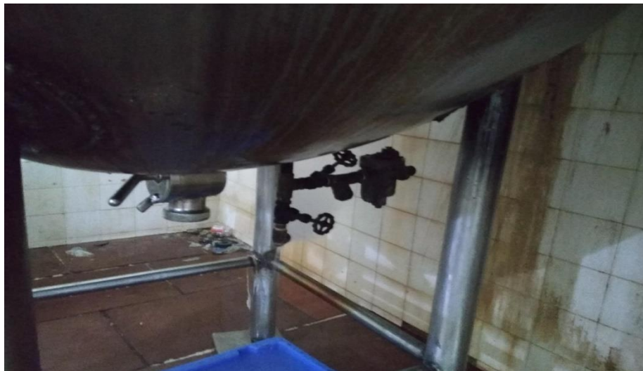
Figure 16: Bucket trap at Curd Section
