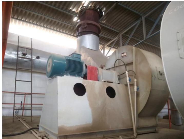
Figure 38: Direct drive blower fan
