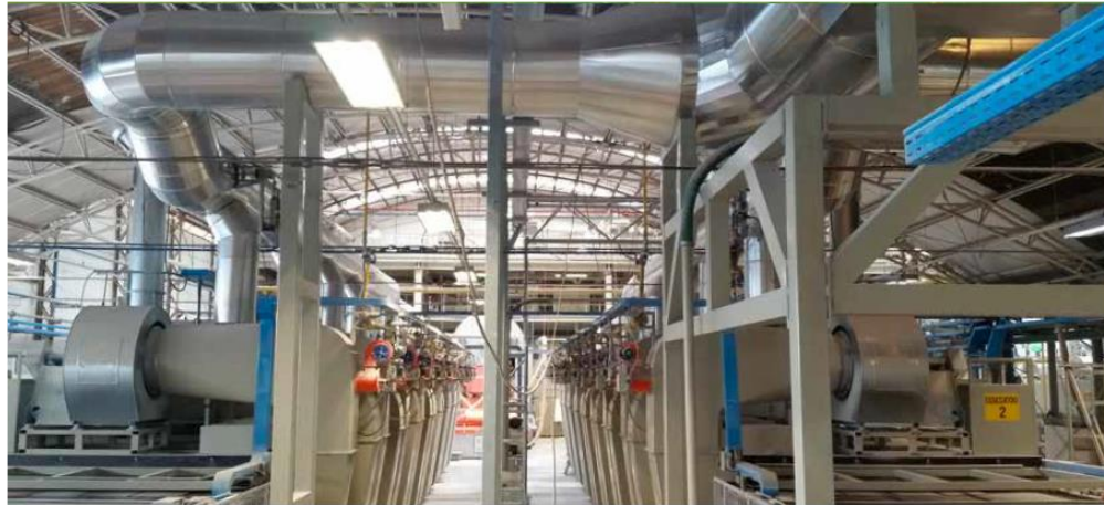
Figure 34: Heat recovery from kiln to dryer
