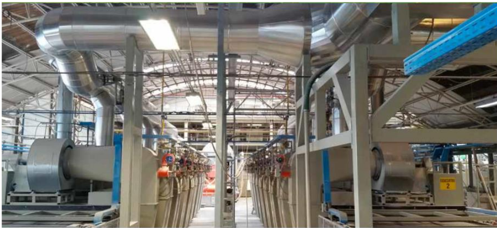
Figure 25: Heat recovery from kiln to dryer
