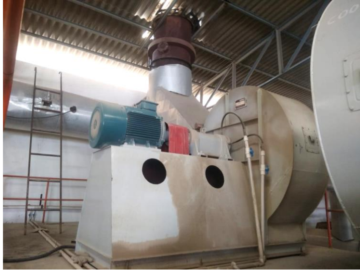
Figure 29: Direct drive blower fan
