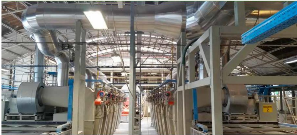
Figure 25: Heat recovery from kiln to dryer
