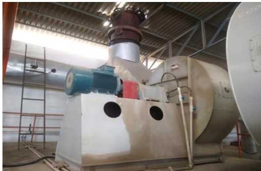
Figure 23: - Direct drive blower fan
