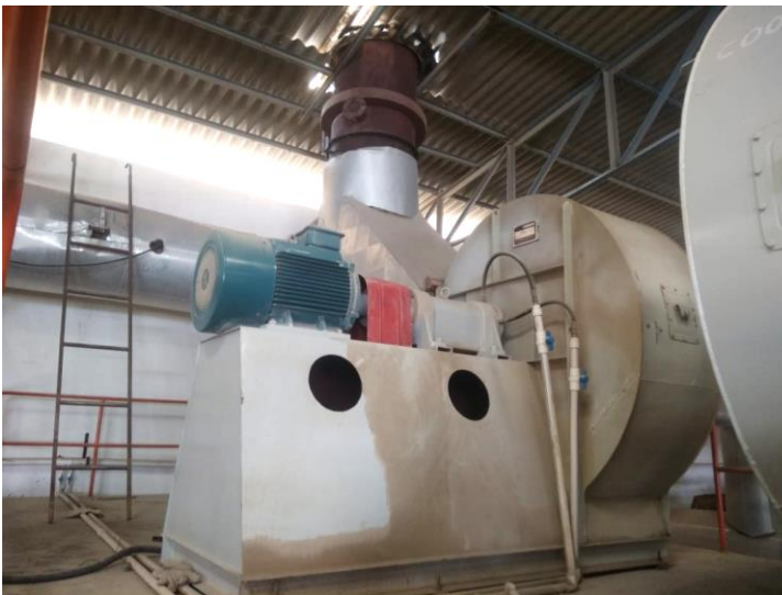
Figure 25: Direct drive blower fan
