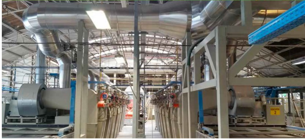
Figure 20: Heat recovery from kiln to dryer
