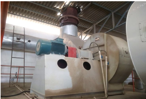
Figure 24: - Direct drive blower fan
