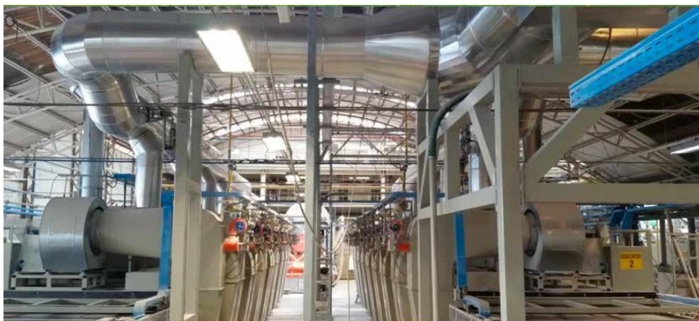
Figure 21: Heat recovery from kiln to dryer
