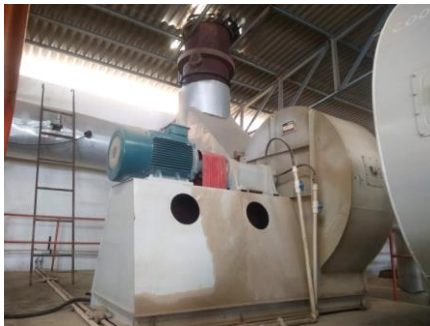
Figure 26: Direct drive blower fan
