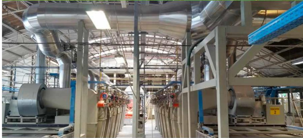
Figure 21: Heat recovery from kiln to dryer
