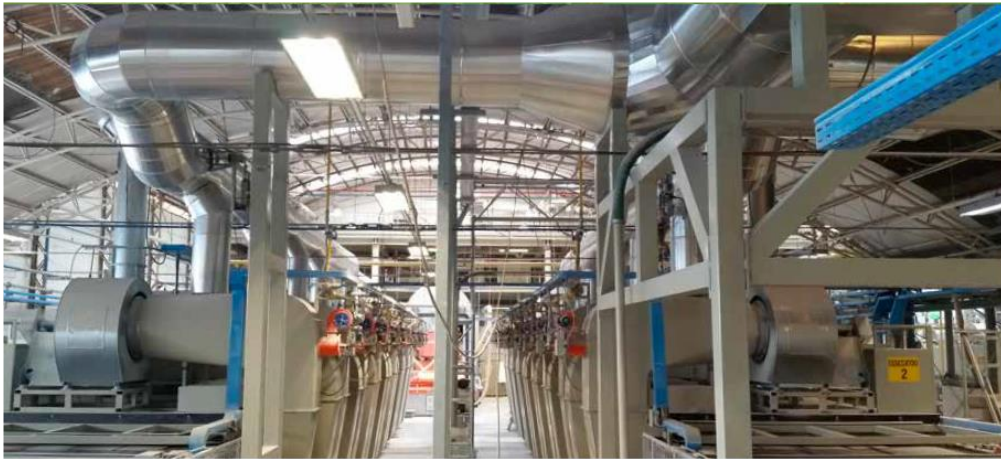
Figure 20: Heat recovery from kiln to dryer
