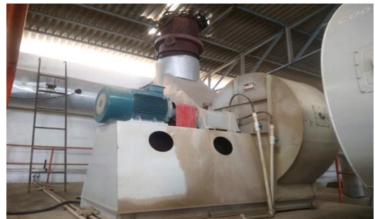
Figure 24: Direct drive blower fan
