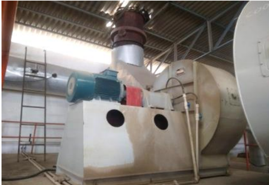
Figure 19: Direct drive blower fan
