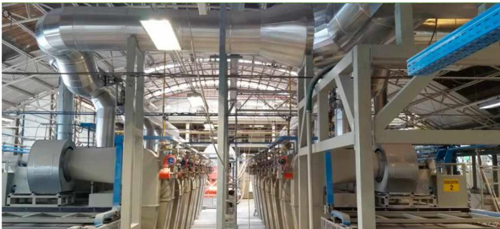
Figure 32: Heat recovery from kiln to dryer
