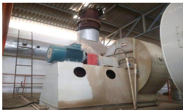
Figure 36: Direct drive blower fan
