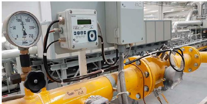
Figure 23: NG consumption monitoring kit
