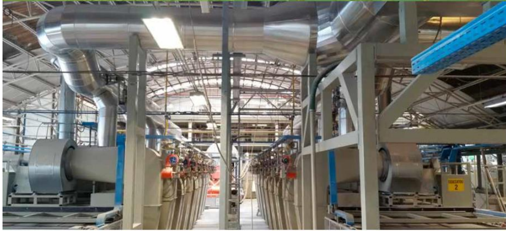
Figure 25: Heat recovery from kiln to dryer
