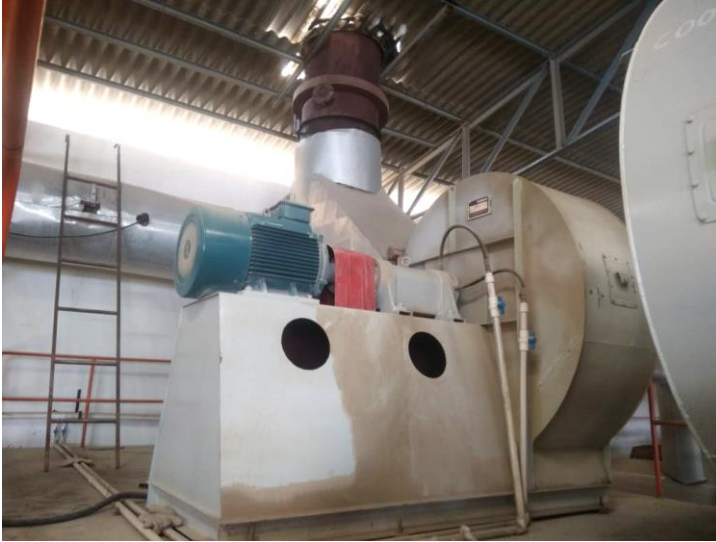
Figure 28: Direct drive blower fan
