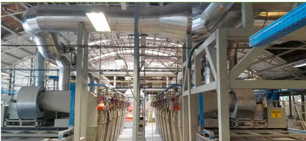
Figure 24: Heat recovery from kiln to dryer
