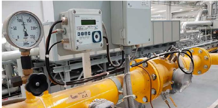
Figure 22: NG consumption monitoring kit
