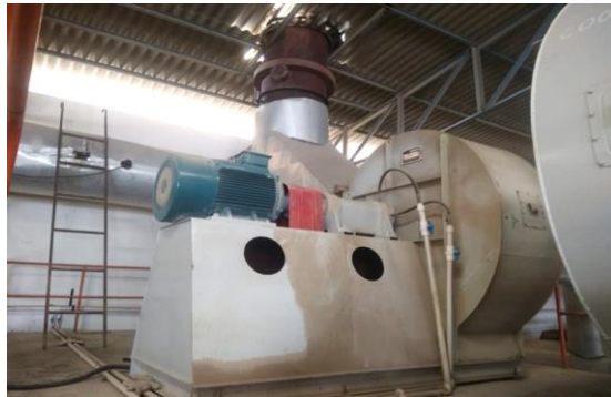
Figure 28: Direct drive blower fan
