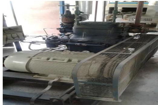
Figure 10: Chiller Compressor
