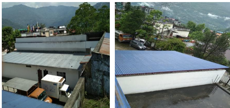
Figure 23: Rooftop area for solar
