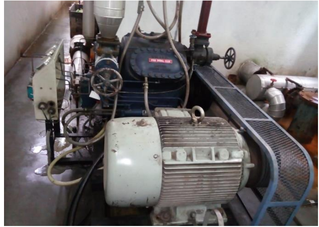
Figure 19: Chiller Compressor
