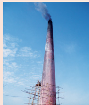
Fixed Chimney BTK
