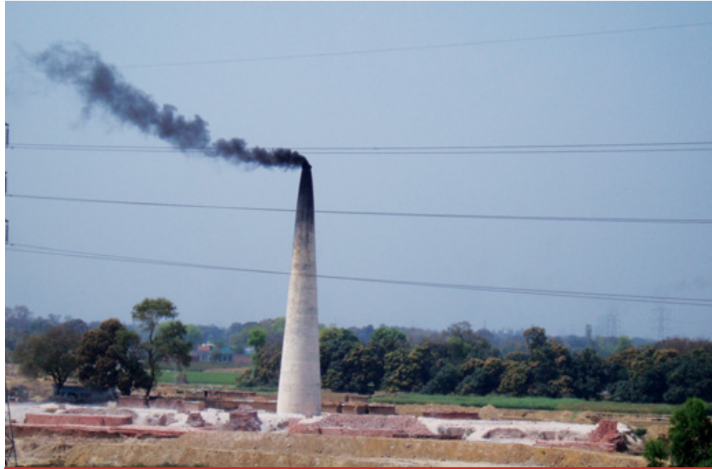
Figure 2 Fixed Chimney Bull's Trench Kiln
