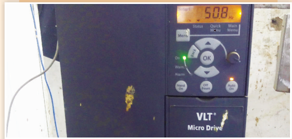
VFD installation at refrigeration compressor motor
