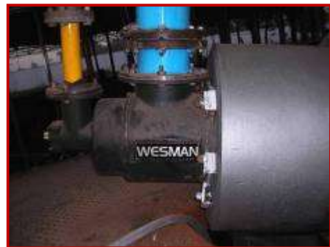
Figure 3.3: High velocity short flame burner for EcoMelt
