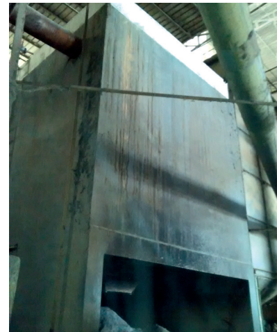
Pollution control cum water preheating system
