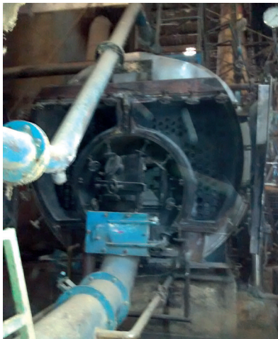
Rice husk-fired boiler
