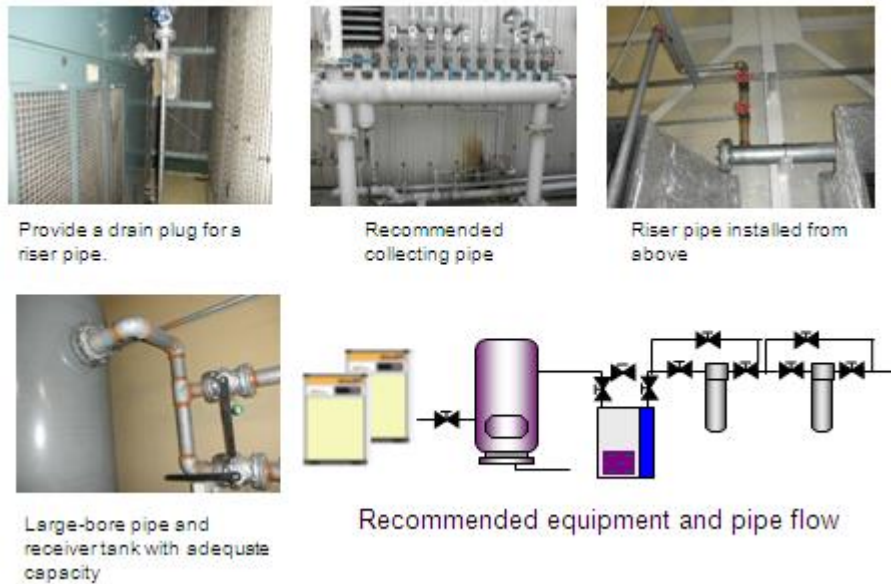
Figure 4.15c: Examples of recommended piping
