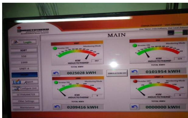
Installation of induction furnace energy monitoring system
