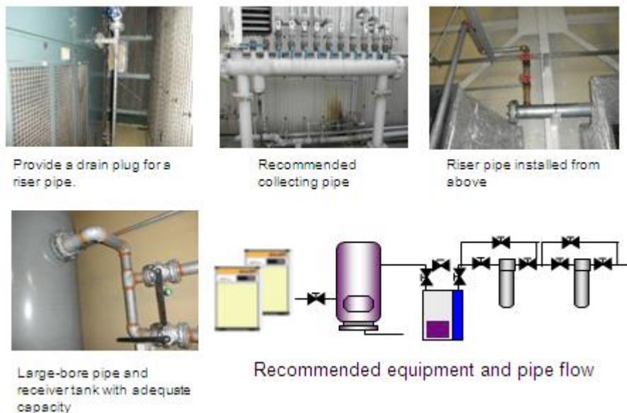
Figure 3.1.5c: Examples of recommended piping
