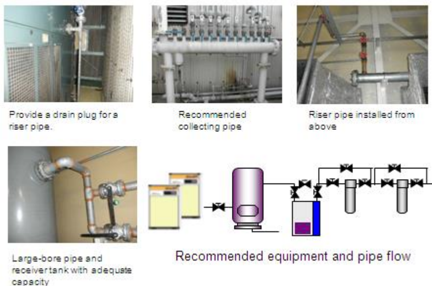
Figure 3.1.5c: Examples of recommended piping
