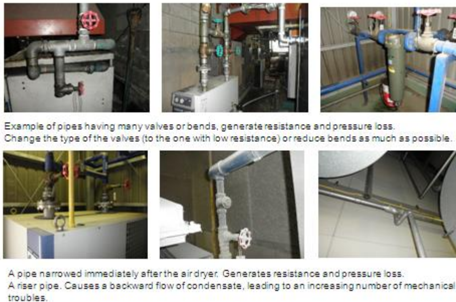
Figure 3.1.5b: Contents of Improvement Measures – Examination of Piping Work
