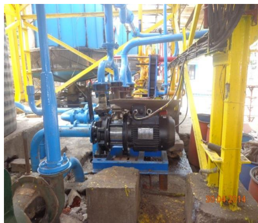
Removal of obstruction to cooling tower air intake and FRP blades
