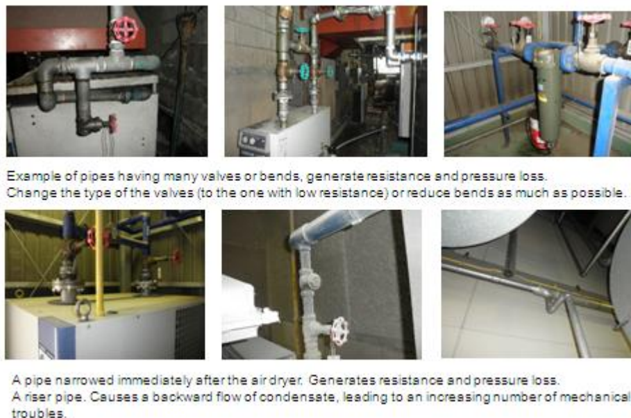
Figure 4.1.5b: Contents of Improvement Measures – Examination of Piping Work
