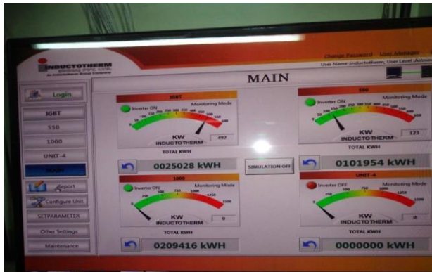
Installation of induction furnace energy monitoring system
