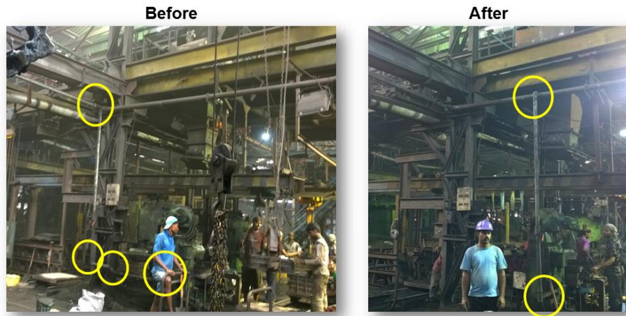
Improvement in compressed air network
