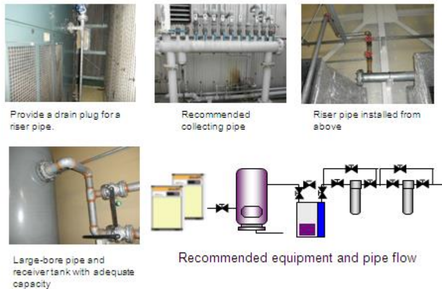
Figure 2.1.5c: Examples of recommended piping
