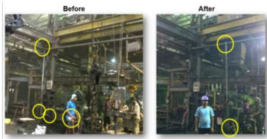
Improvement in compressed air network
