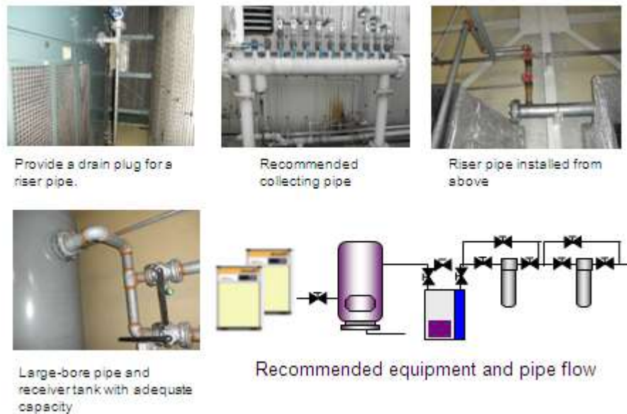
Figure 3.1.5c: Examples of recommended piping
