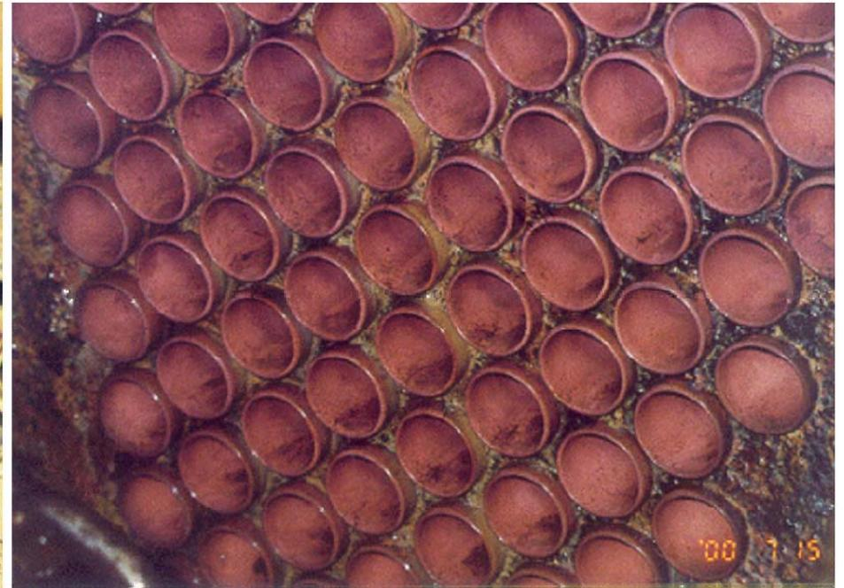
Tube after installation of Auto ball cleaning system
